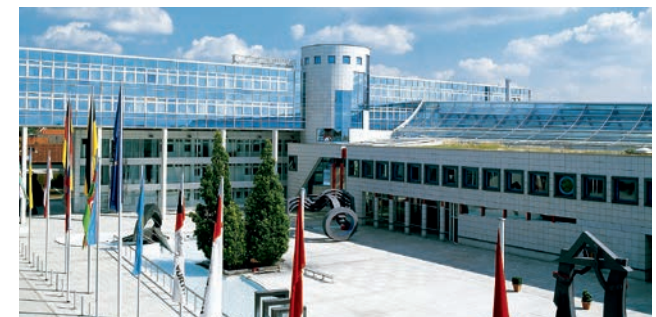
Würth administration building in Künzelsau
