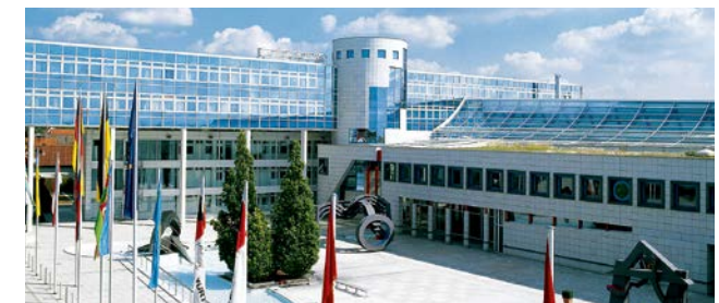
Würth administration building in Künzelsau
