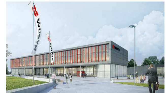
The polygonal and expressive shape of the building underpins its importance as an innovation center.
