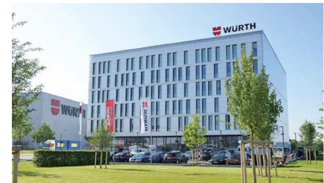
New branch office and administration building at Adolf Würth GmbH & Co. KG in Künzelsau-Gaisbach
